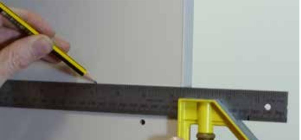
11. Using the “SPACE TOWER marking template”, place over the centre lines and place a mark at the “RUNNER” positions as marked on the template. Do this for all of the runner positions.
